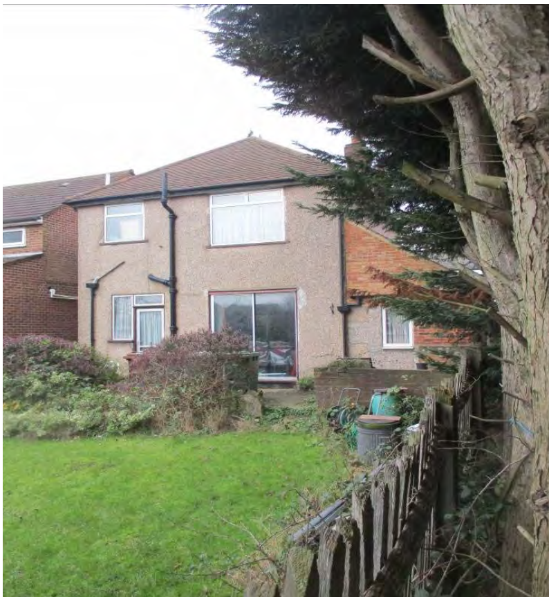
Rear of no. 7
