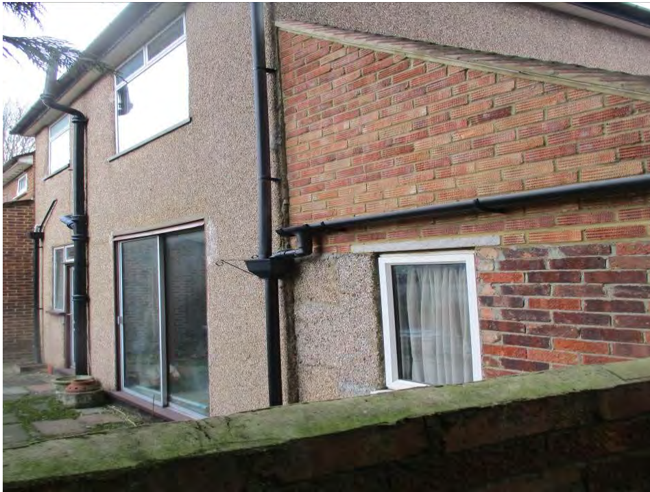
Rear of garage adjacent to boundary with no.9
