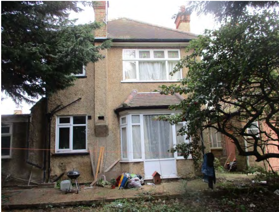
Rear Elevation of no. 9
