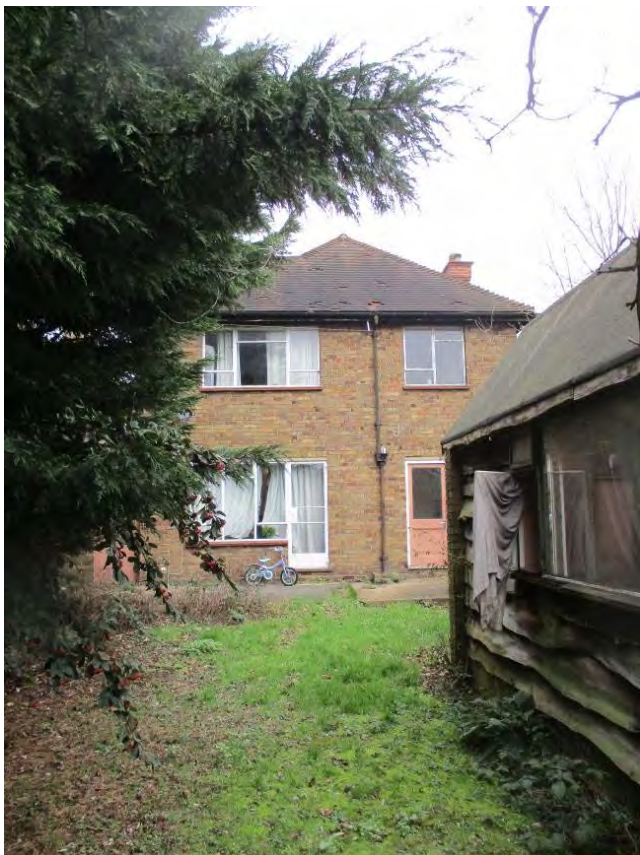
Rear of no. 11
