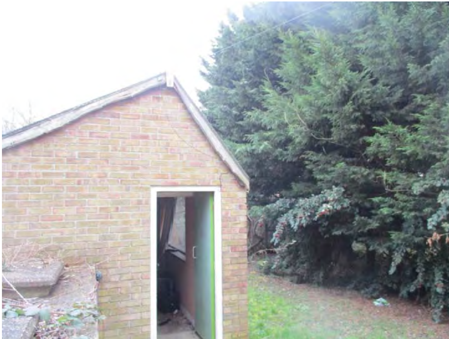
Rear outbuilding at no. 11
