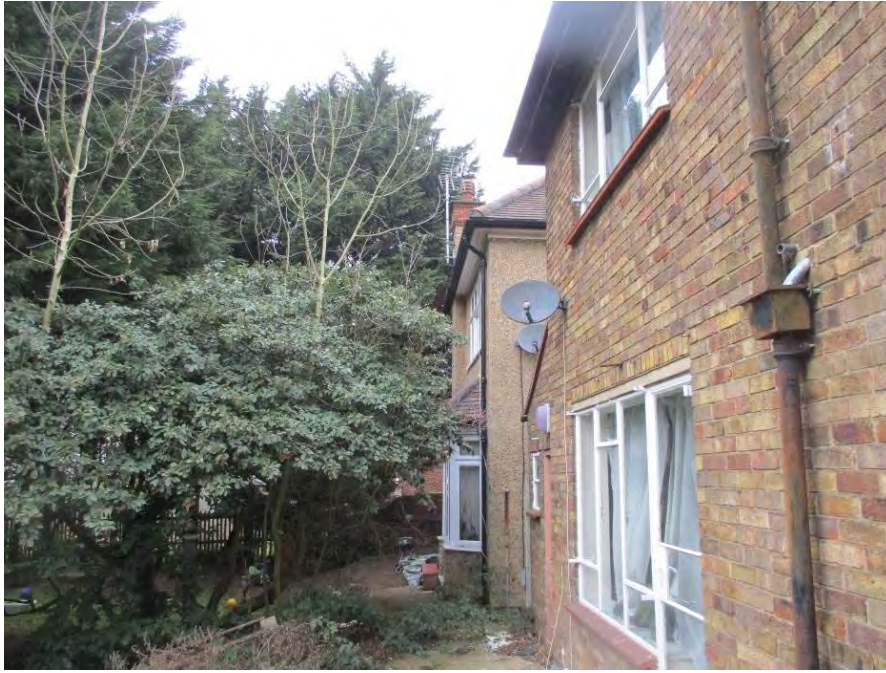
Rear elevations of no. 9 and 11
